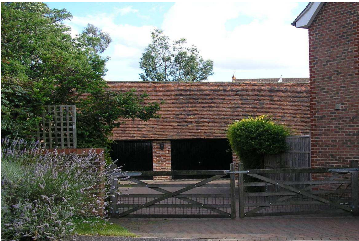
Modern housing at Moat Farm incorporating former agricultural building as garaging.
