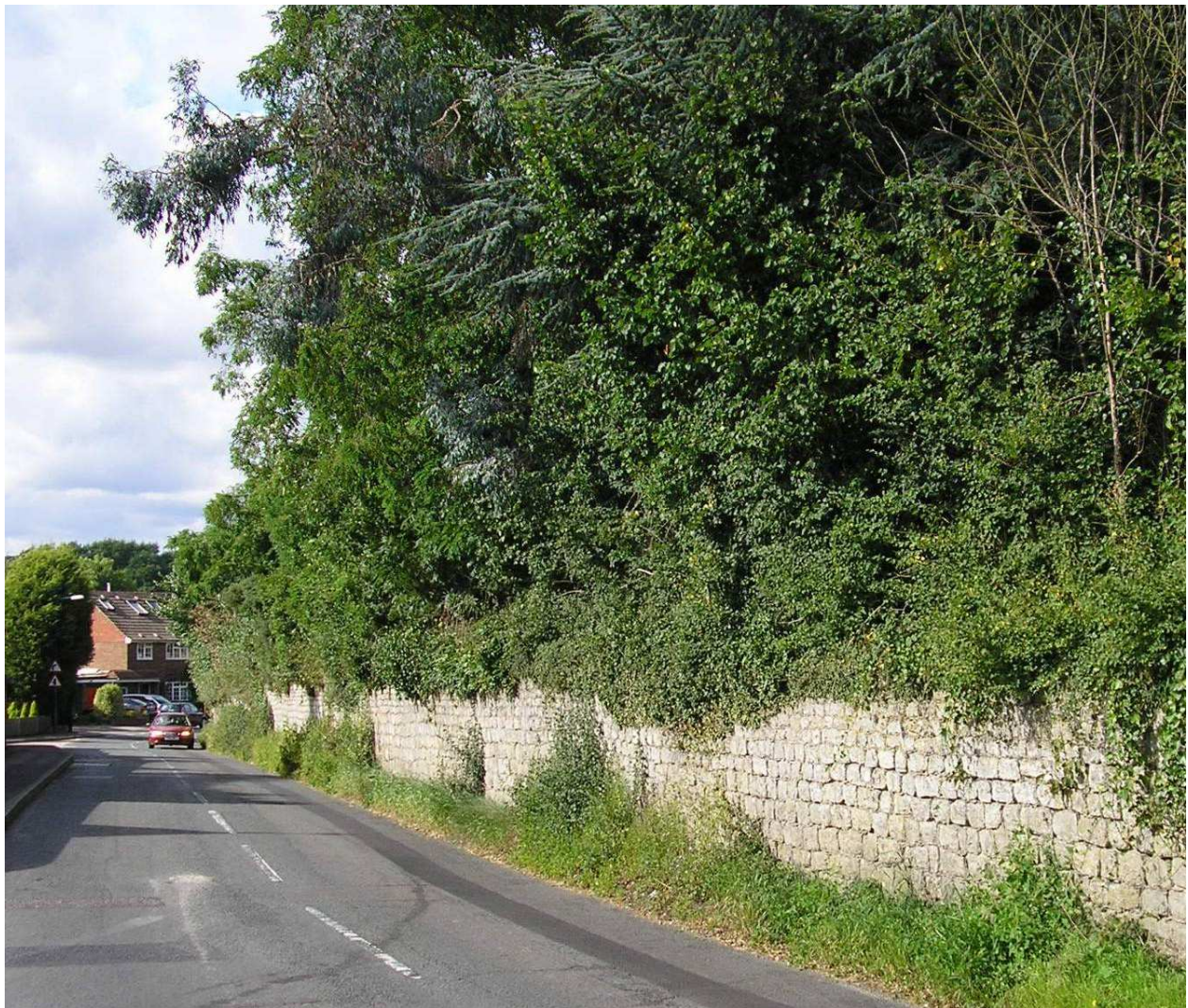
An important feature of Homedean Road is the planting and this long coursed ragstone wall.
