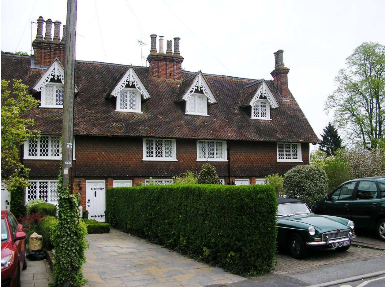
Former estate cottages, 43-53 High Street
