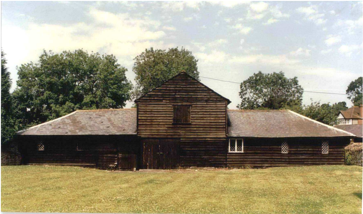
The symmetrical elevation and 19 th Century lattice windows indicate a considered design for this former agricultural building perhaps reflecting its origins as an Estate building
