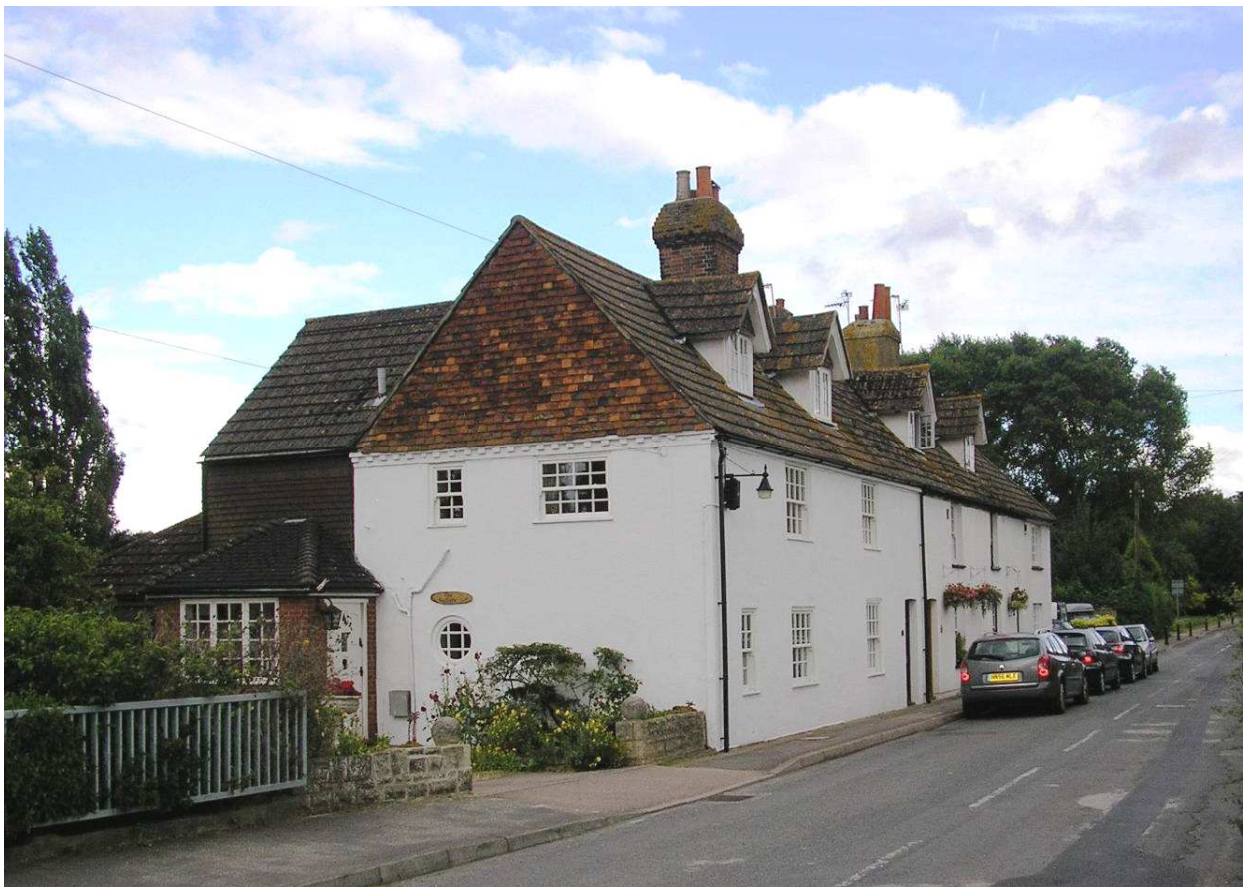
Historic cottages in Chevening Road
