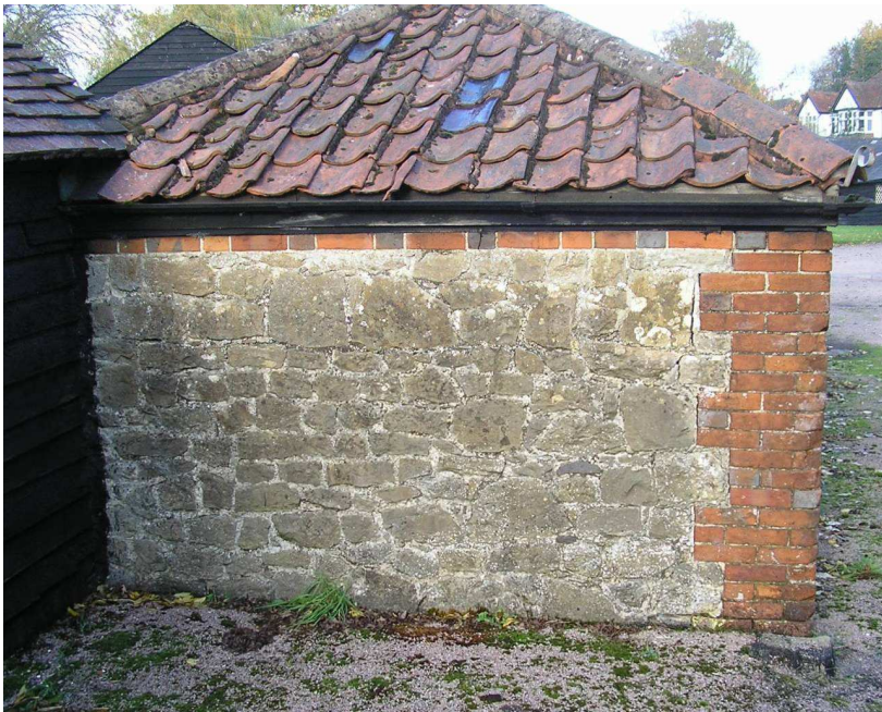
Simple vernacular detailing.
