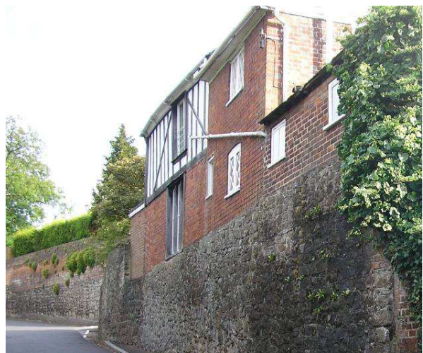
Soil pipe on Bank House
