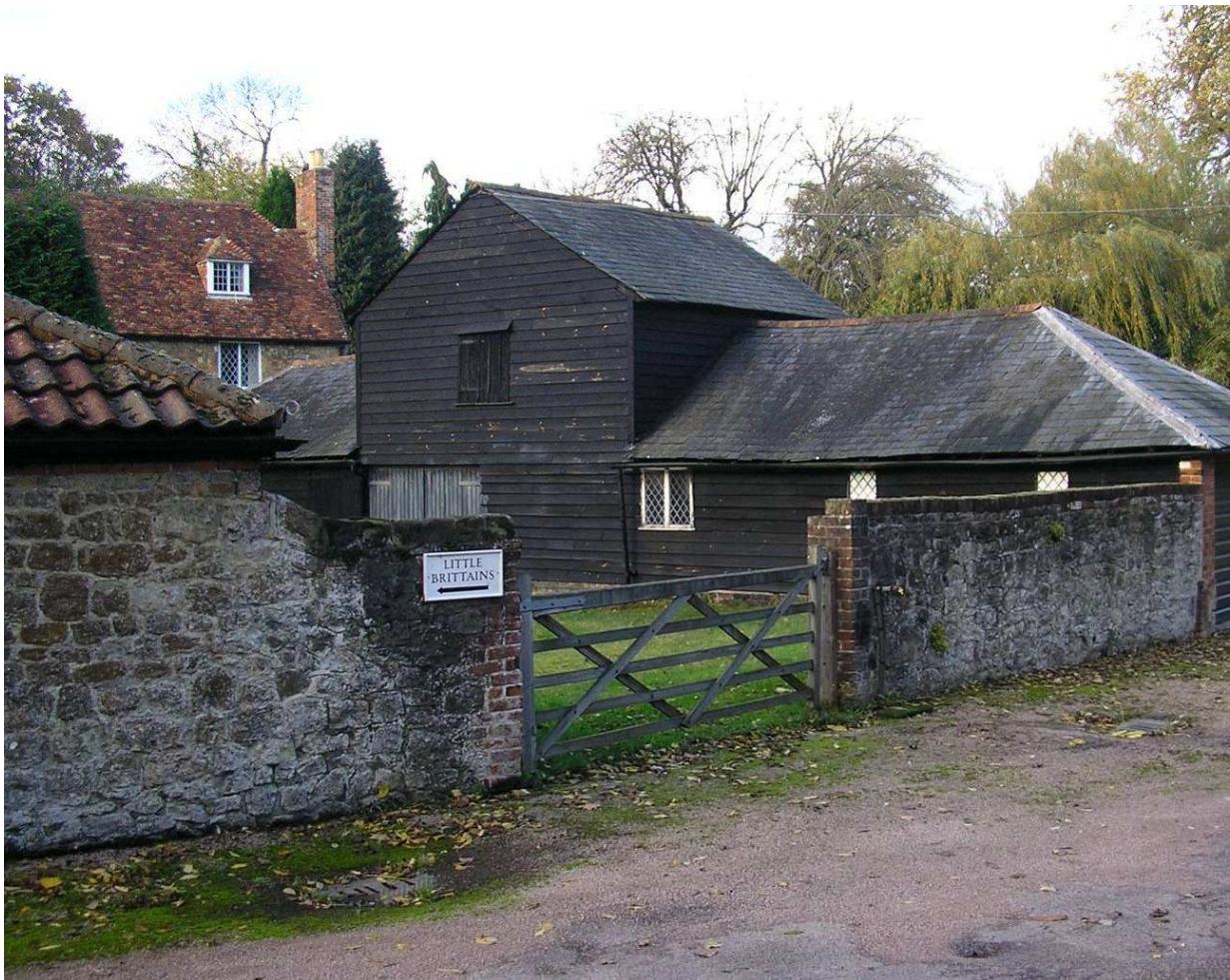
The subtle mix of materials and retention of informal building groups adds to the character of Brittain's farmstead.
